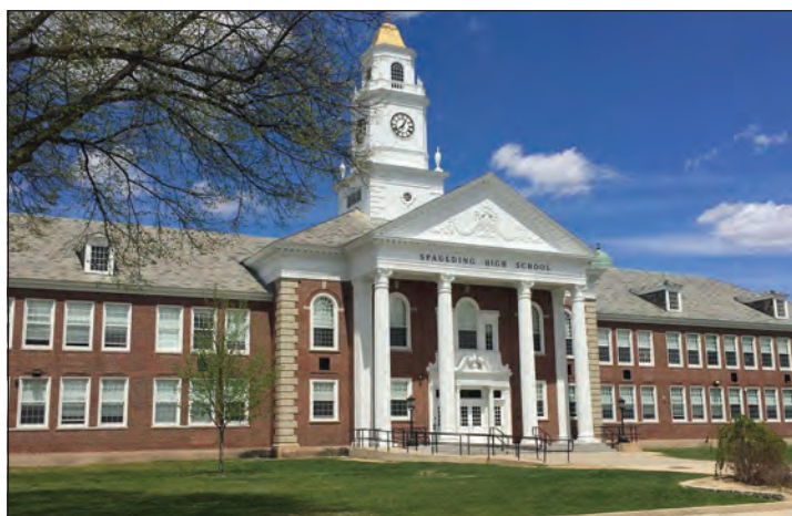
Spaulding High School sprinkler & fire alarm upgrade
