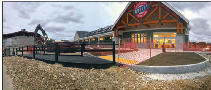
NH Liquor Commission's Outlet Store featured post and beam clerestory over the sales floor.
